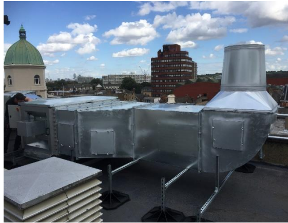
External Plant Deck
